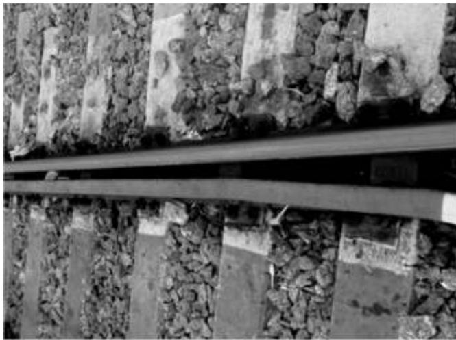
**P&C sleepers with Rail screw used on diamond crossing**
